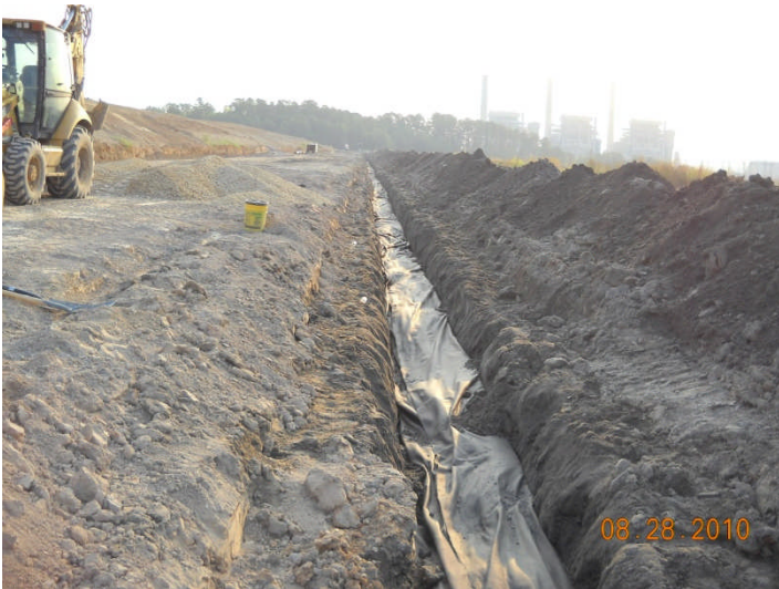
MSI, toe drain installation, PDP 3
