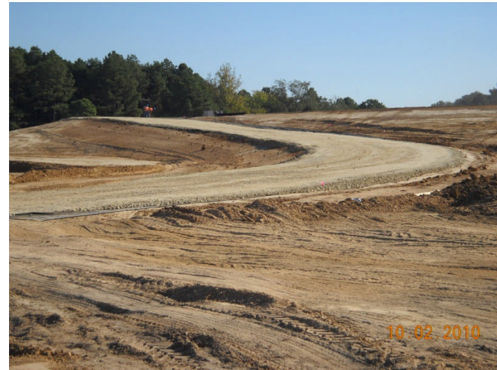
MSI, access road construction, NW PDP 1
