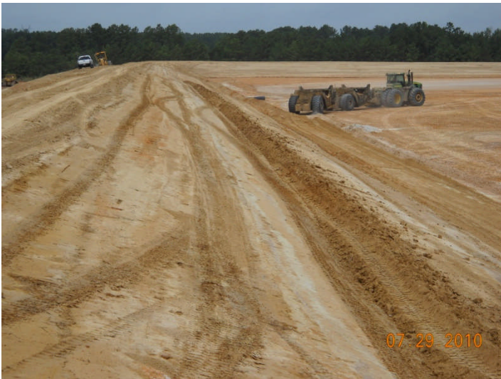
MSI, interior berm structural fill grading, PDP 3
