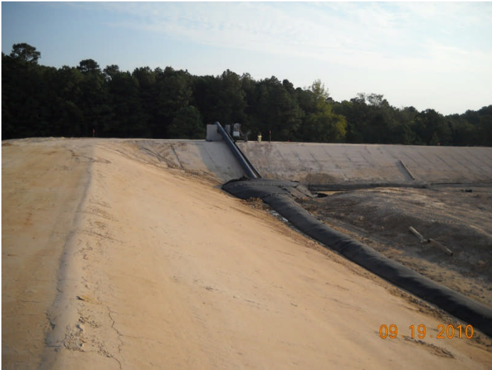
MSI, completed leachate sump, NE PDP 1
