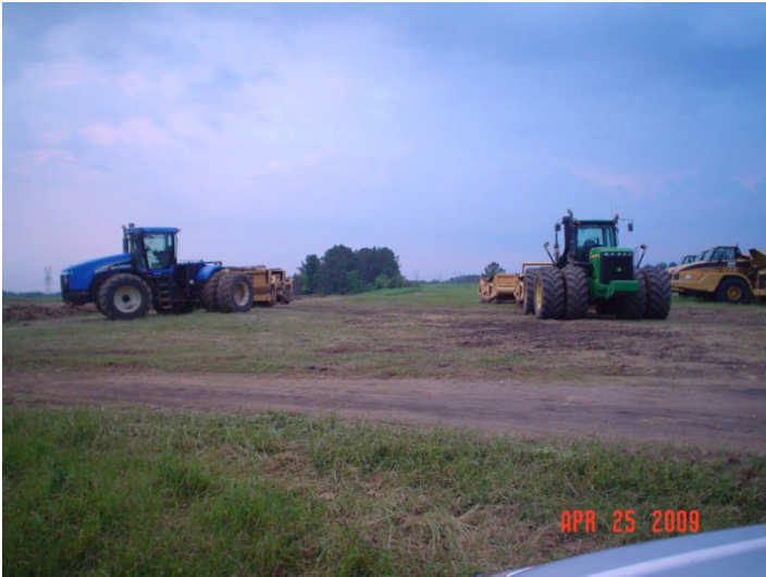
Pickett, mobilization, staging area
