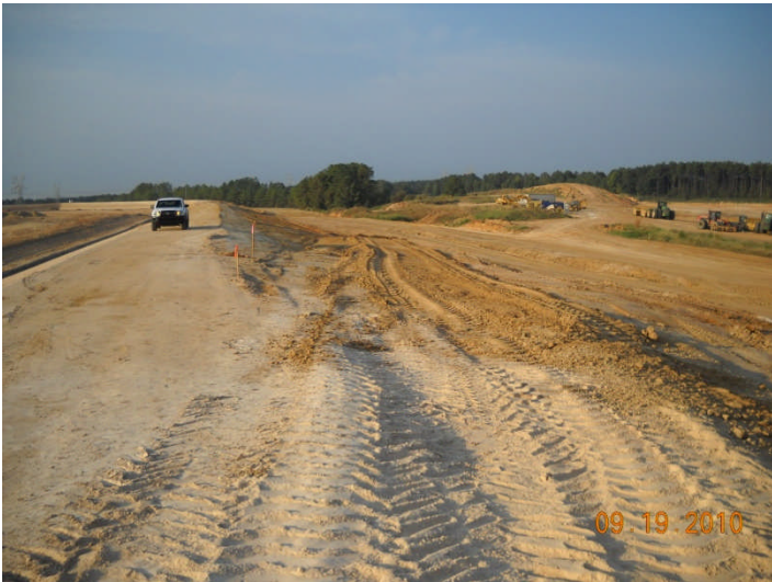
MSI, access road construction, NW PDP 1
