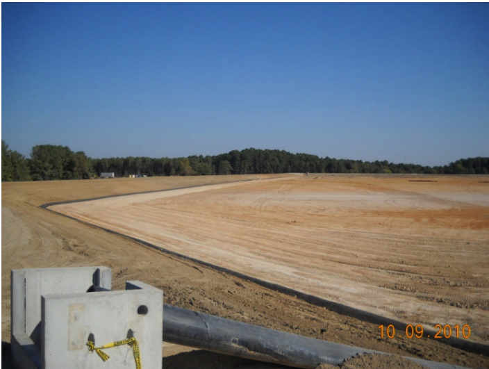
MSI, final grading, SW PDP 3 looking North
