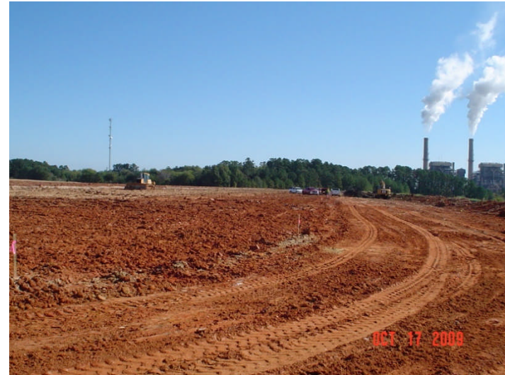
Rodman, establishing sub-grade and perimeter, PDP 3
