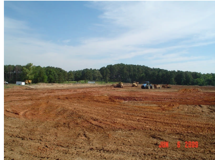
Pickett, placing first lift clay liner, NW PDP 1-2
