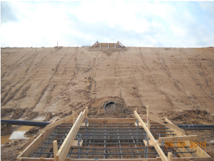
MSI, decant pads preparation, PDP 3
