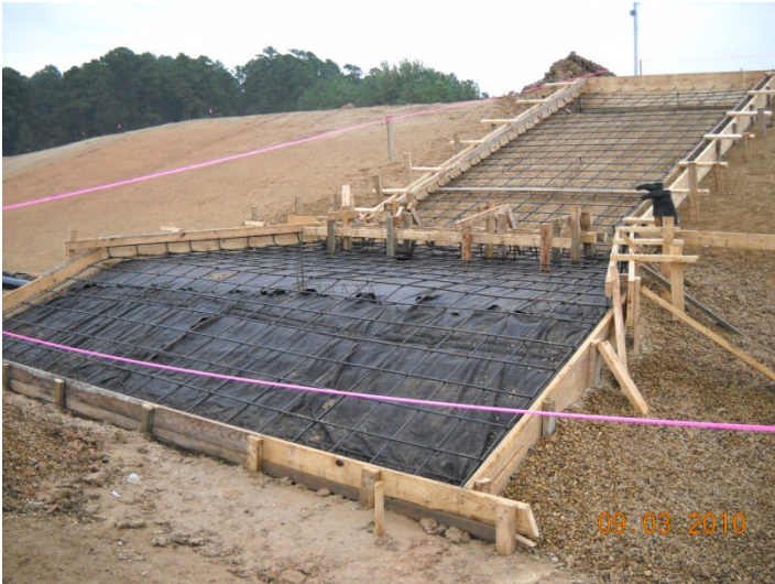
MSI, slurry channel preparation, PDP 1
