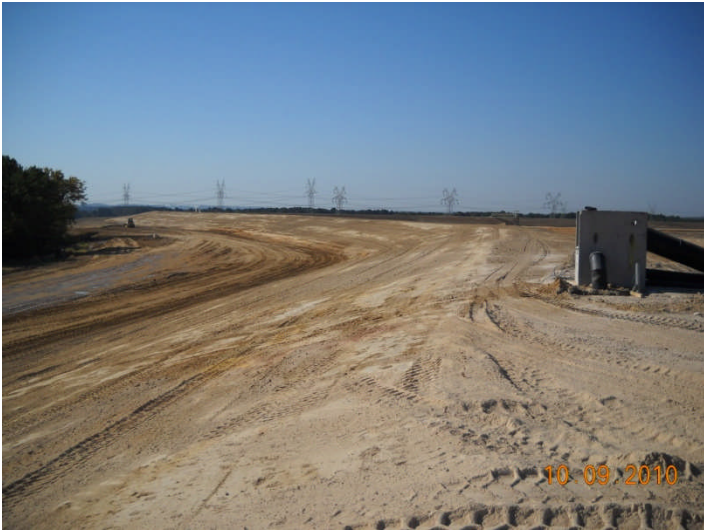
MSI, final grading, NE PDP 1 looking South
