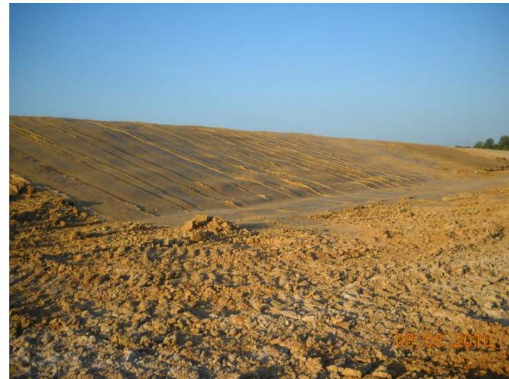
MSI, interior slope liner processing, PDP 3
