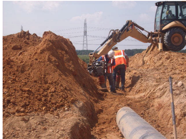
MSI, berm penetration and compaction, PDP 3
