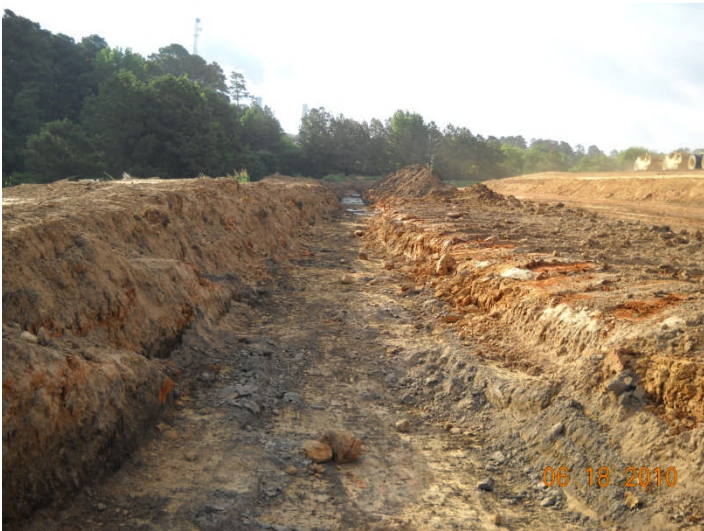
MSI, clay liner tie-in, PDP 1
