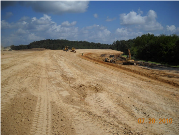
MSI, exterior berm grading and clay liner tie in, SE PDP 2-3
