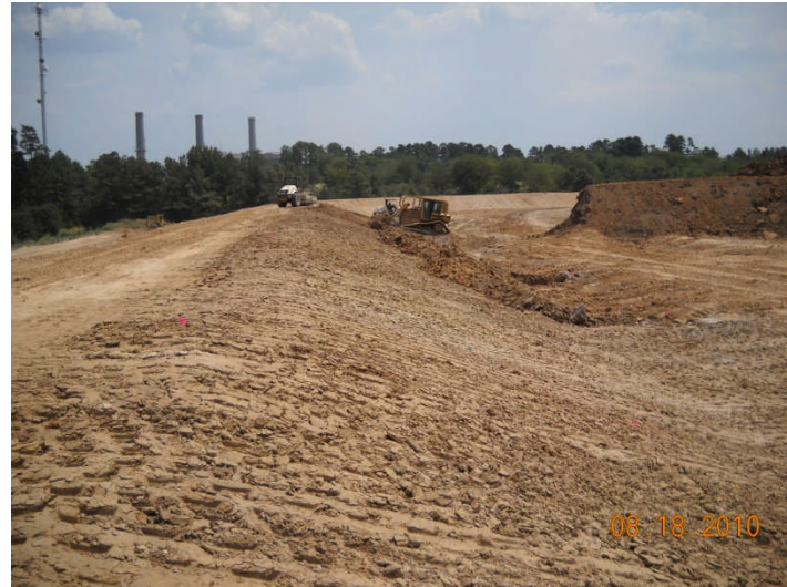
MSI, interior slope liner placement and processing, PDP 1
