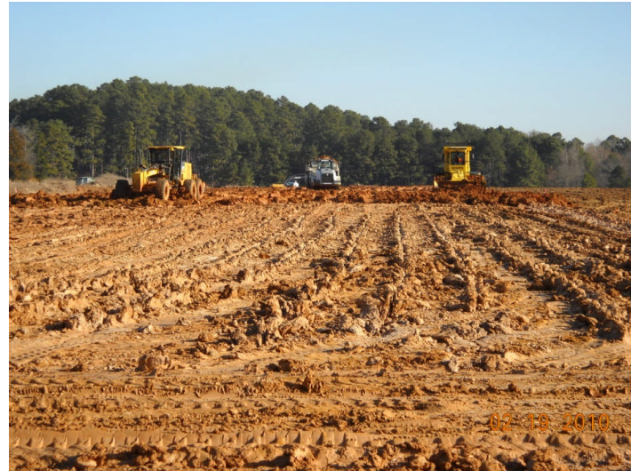
Rodman, liner placement and processing, PDP 1-2
