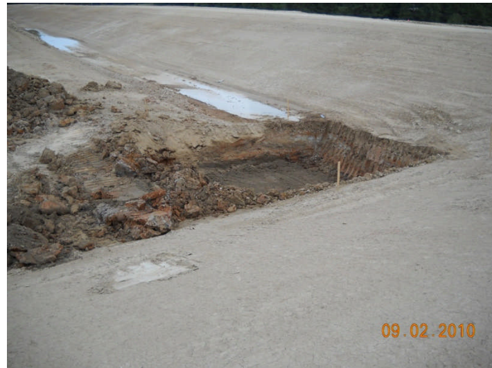
MSI, leachate sump preparation, PDP 1
