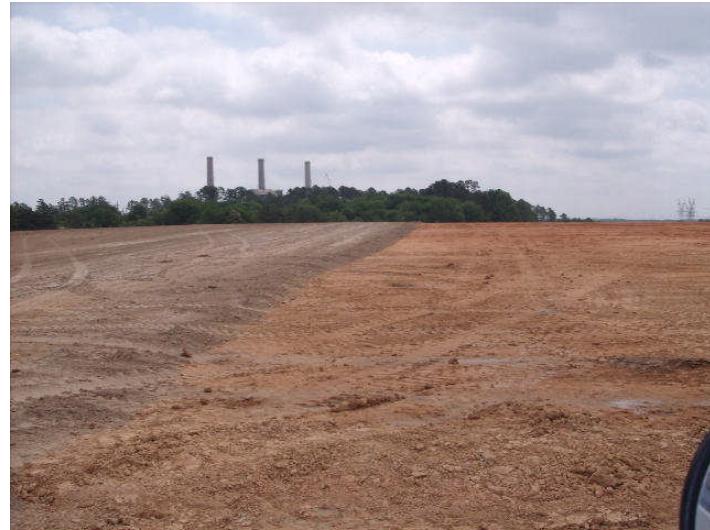
MSI, protective cover placement, Eastern PDP 2
