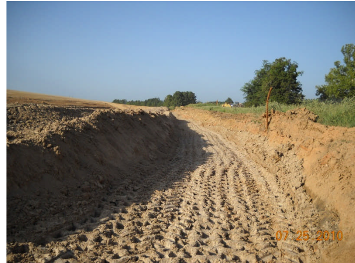
MSI, clay liner tie in compaction, NW PDP 1
