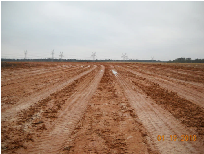
Rodman, liner compaction, Eastern PDP 1-3
