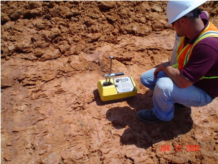
Nuclear density and moisture testing
