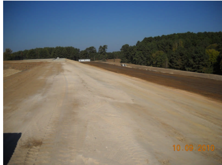
MSI, final grading, NE PDP 1 looking West
