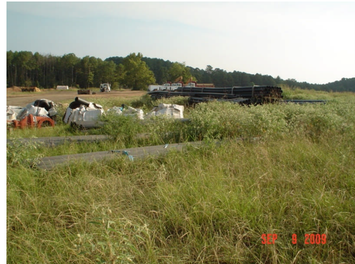
Pickett, de-mobilization, staging area
