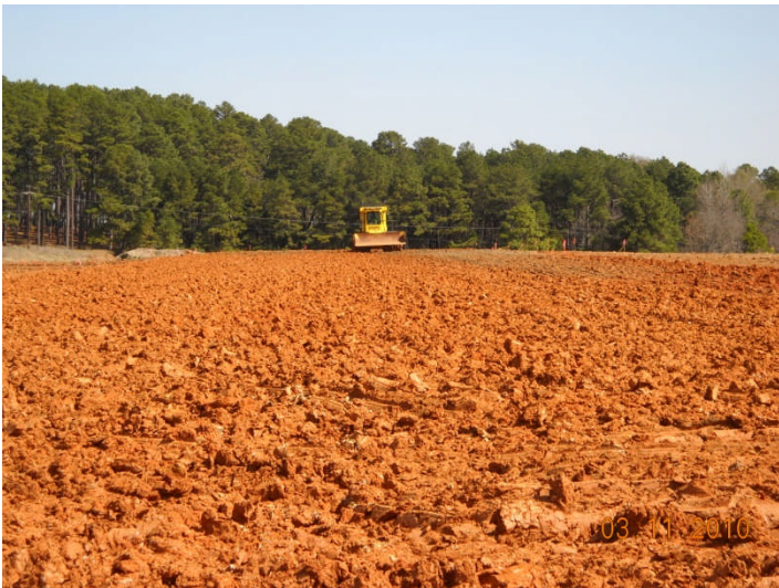
Rodman, berm structural fill processing, Western PDP 1-2
