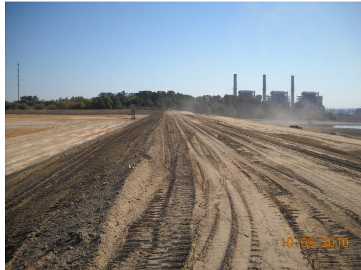
MSI, final grading, SW PDP 3 looking East
