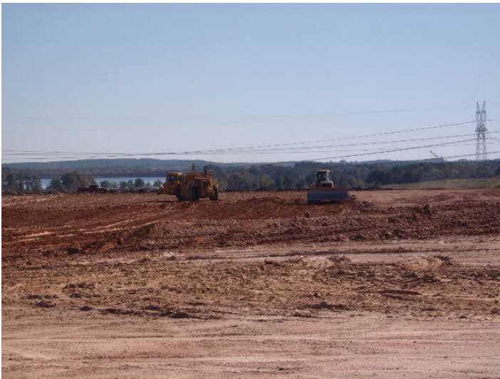
Rodman, establishing sub-grade and perimeter, PDP 2-3
