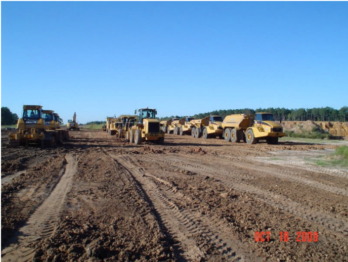
Rodman, mobilization, staging area
