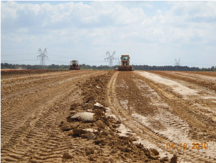
MSI, liner grading and berm processing, SE PDP 2-3
